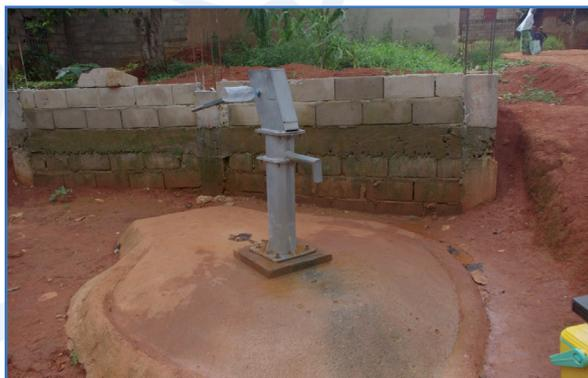
Figure 4: Well maintained dug well with a hand pump used by 400 people as drinking water supply
