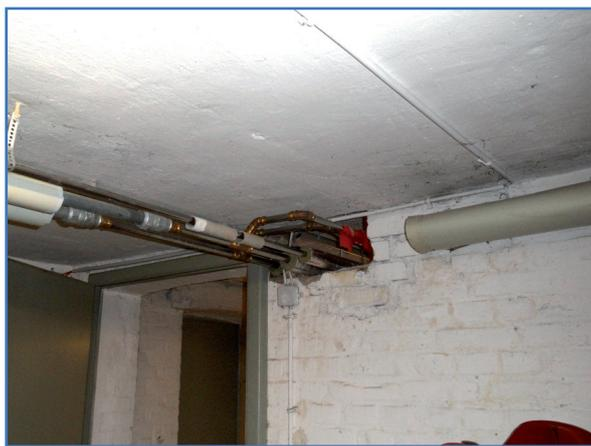
Figure 2: Insufficient insulation of the piping
