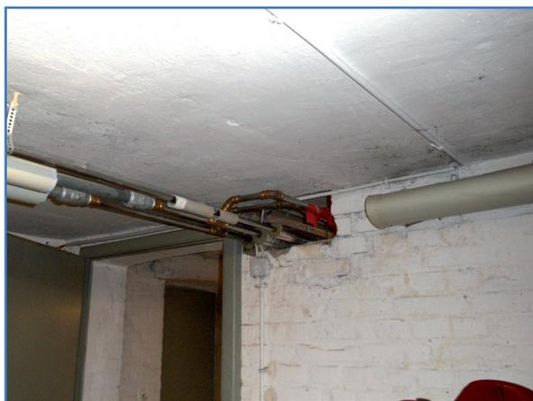
Figure 2: Insufficient insulation of the piping
