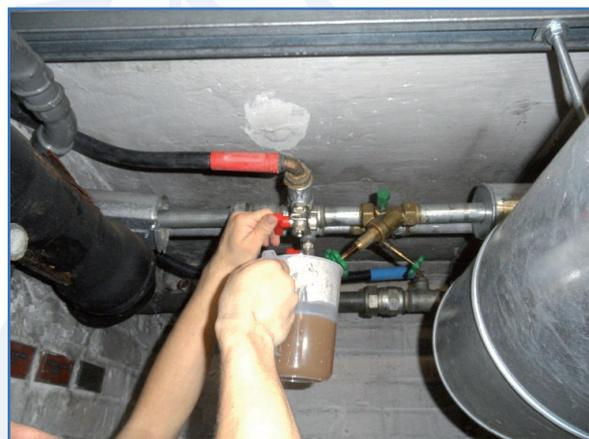
Figure 1: Discoloration of water taken from the drinking water pipeline
