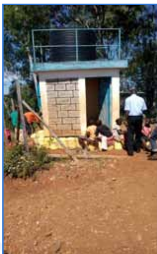
Figure 3: A communal water kiosk (Source: J. Wasonga)
