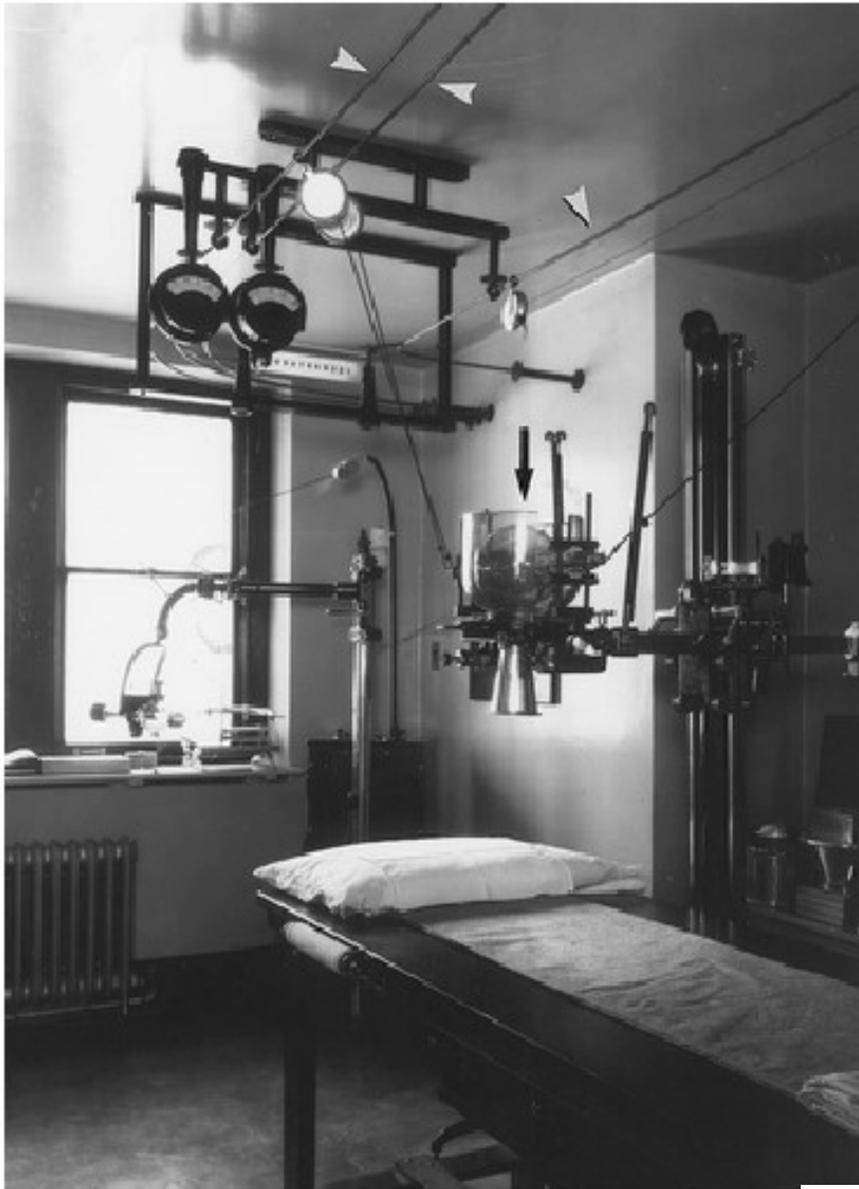
An x-ray examination room (Mayo Clinic, Rochester, Minnesota, circa 1925) with bare high-voltage cables (arrow-heads) and little shielding of the x-ray tube (arrow)
