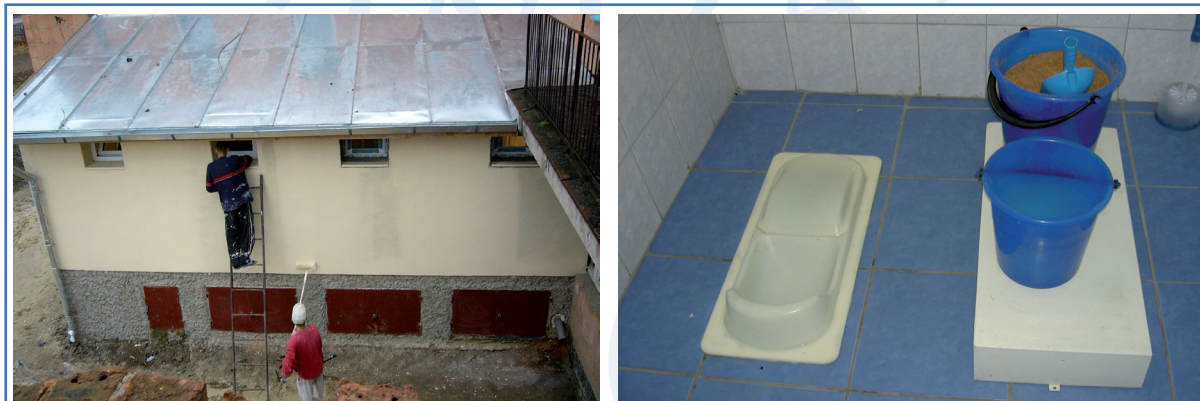
Figure 3: Exterior and interior of the double vault dry UD toilet facility, built in conjunction with the school for 160 pupils: hygienic, safe and easily accessible without leaving the school.
