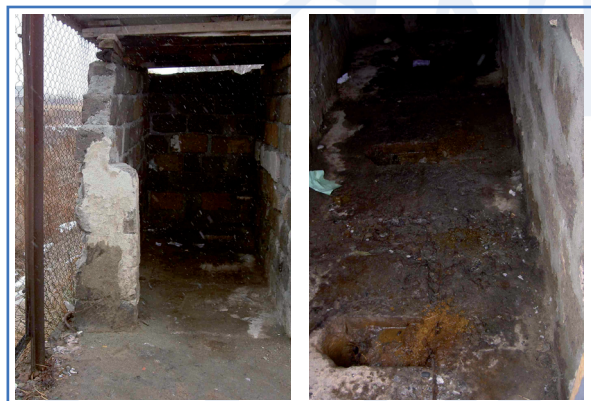
Figure 2: Exterior and interior of a latrine for 360 pupils: no privacy, unhygienic, cold and slippery during wintertime Source: WECF
