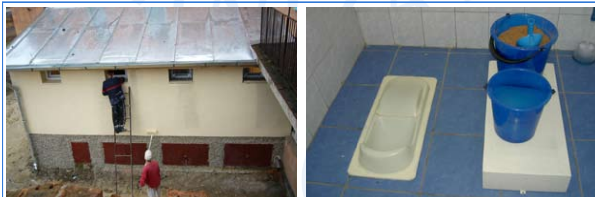
Figure 3: Exterior and interior of the double vault dry UD toilet facility, built in conjunction with the school for 160 pupils: hygienic, safe and easily accessible without leaving the school.
