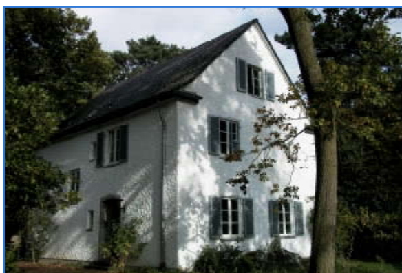
Figure 1: Side building of the Institute for Hygiene and Public Health with the office of the WHO CC Bonn
