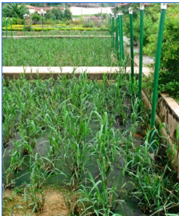
Figure 2: Constructed wetland Source: IHPPH
