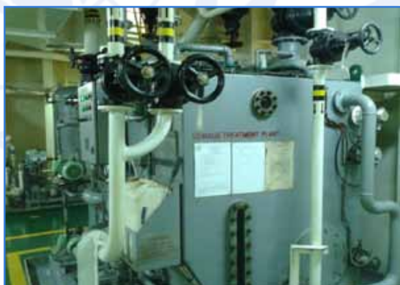
Figure 3: Sewage treatment plant on a ship Source: Kristina Militzer
