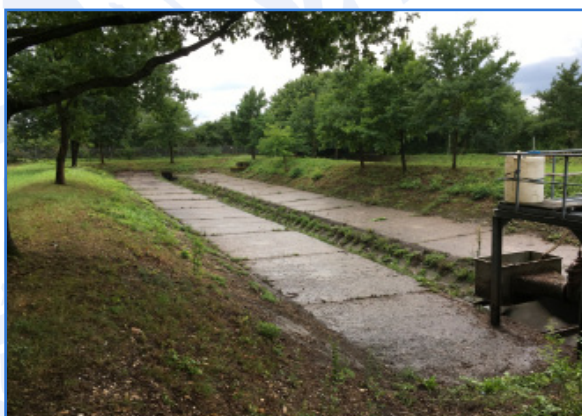
Figure 3: Sampling point for the analysis of stormwater discharge from a separation sewer system at the outlet of a rainwater retention basin (Source: Erftverband)
