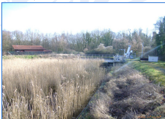
Figure 1: Retention soil filter (Source: Ertverband)
