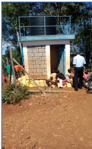
Figure 3: A communal water kiosk (Source: J. Wasonga)
